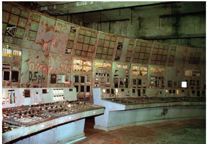
Chernobyl nuclear power plant control room - 25 years after 1986 accident. Photo: The Telegraph.
